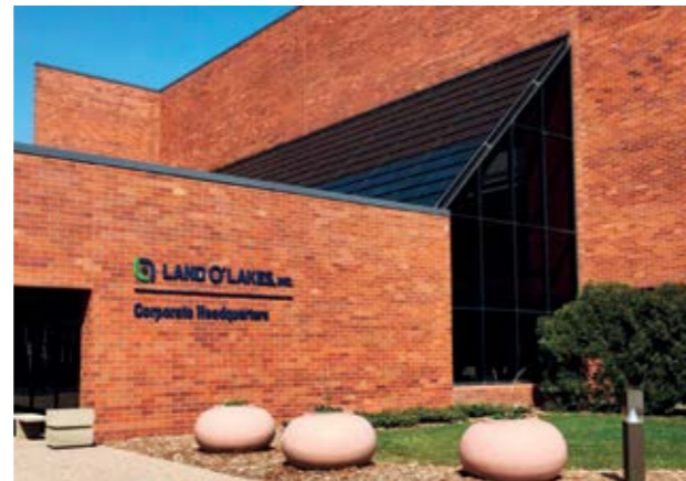
Abb. 58: Office building, retrofit and energy savings of 15%.
