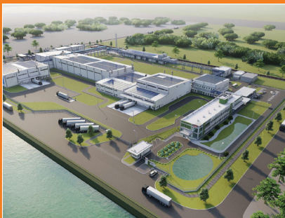
NEW TESA HAI PHONG FACTORY Hai Phong City
