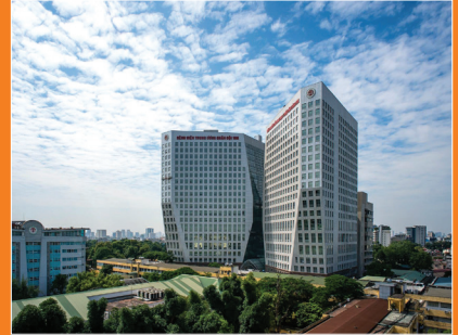
THE CENTRAL HOSPITAL ARMY 108 Ha Noi City
